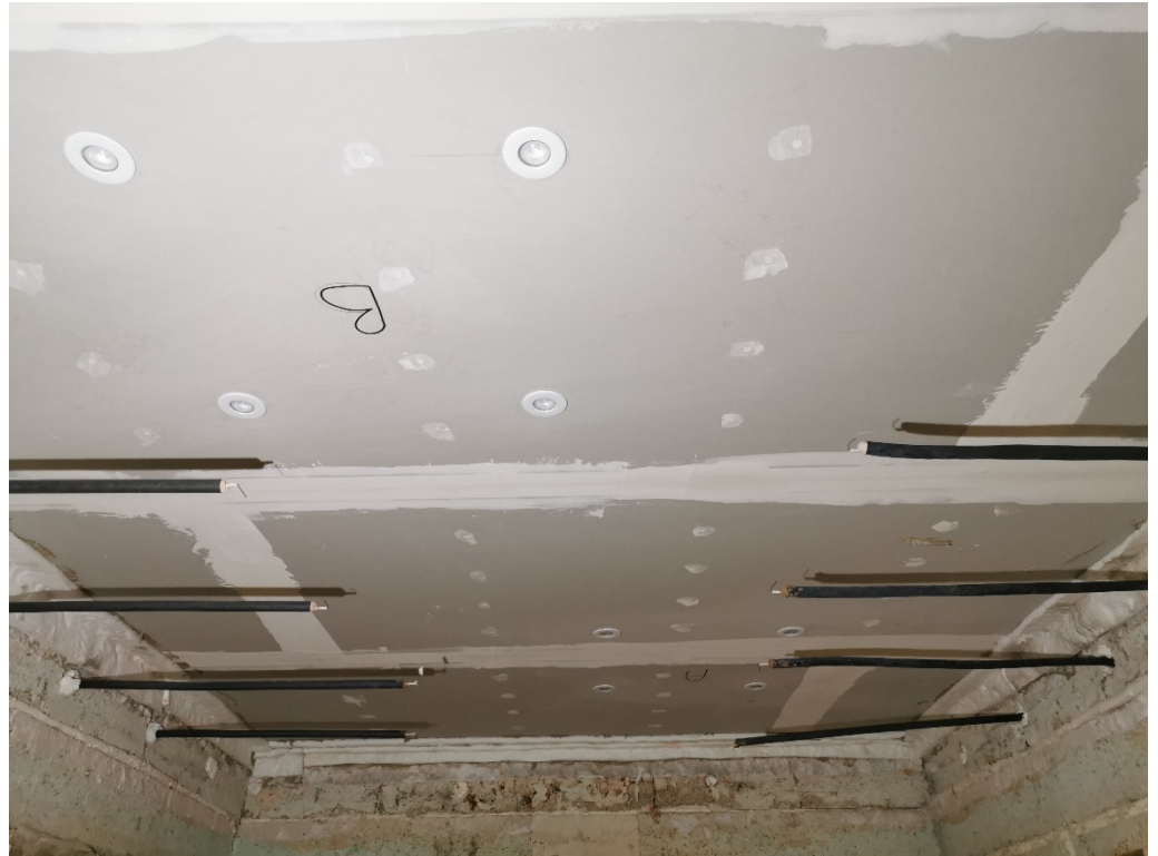
The exposed face of the floor assembly prior to test
