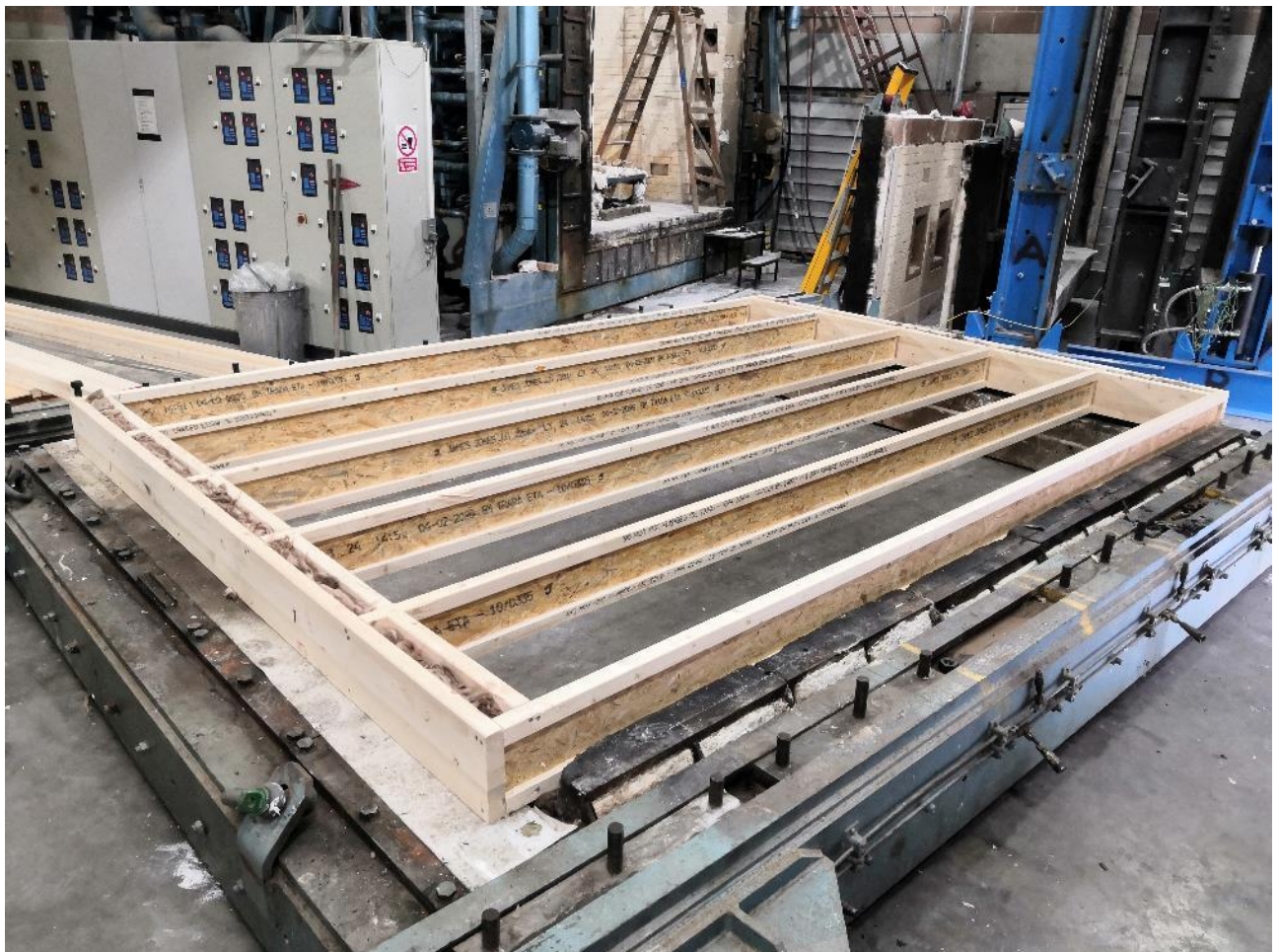
Photograph 1 – Overall view of the completed frame
