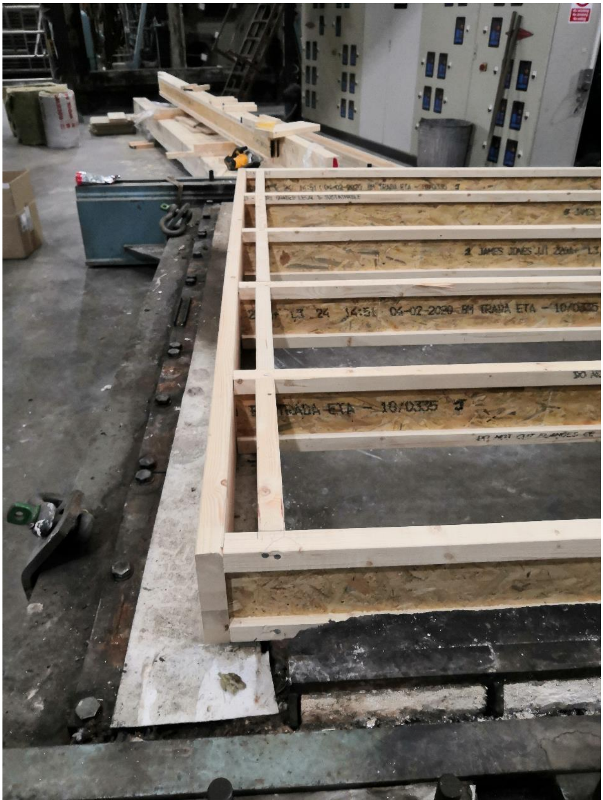
Photograph 2 - Detail of the sample frame. Note the placement of the frame elements and the cavity formed between the rim board and the timber blocks (photo taken before the cavity being filled with glass mineral wool).
