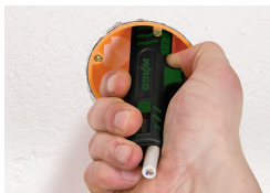
Stripping a cable sheath.
